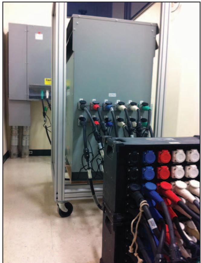
Figure 7 – Mirus International Dual Output HMT Autotransformer equipped with optional Camlok connectors.
